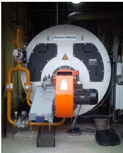
Figure 1 : 1 st installed Modulo + in VALPACO
